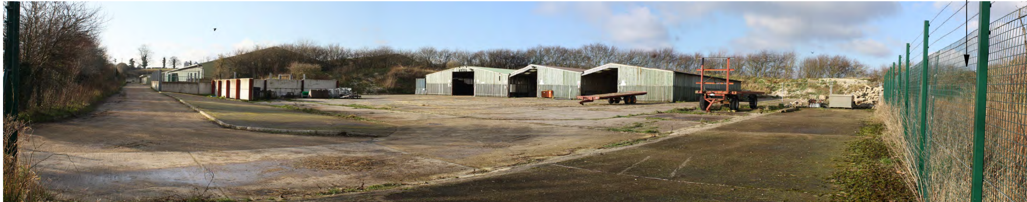
SITE APPRAISAL PHOTOGRAPH A: AREA A
